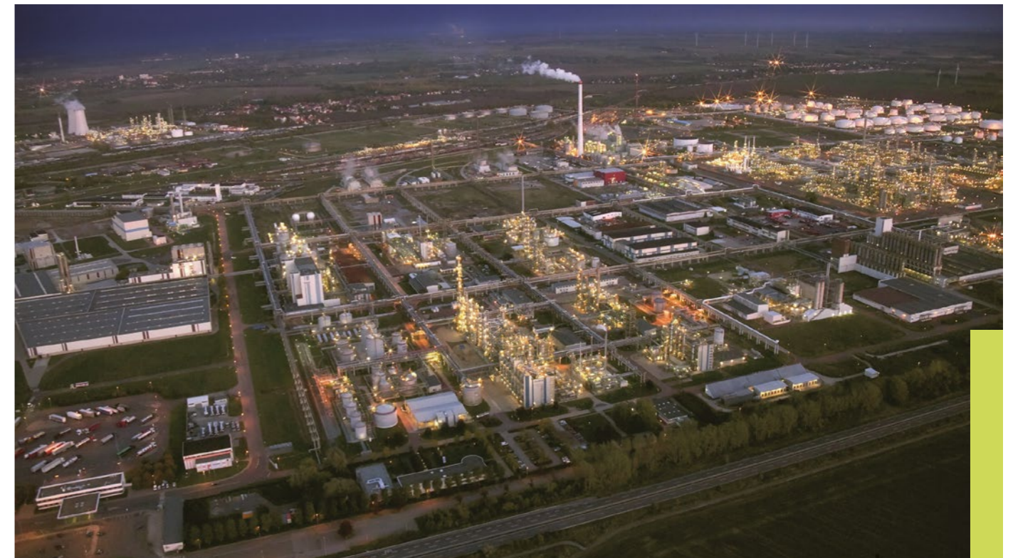
Leuna chemical site © Linde GmbH
